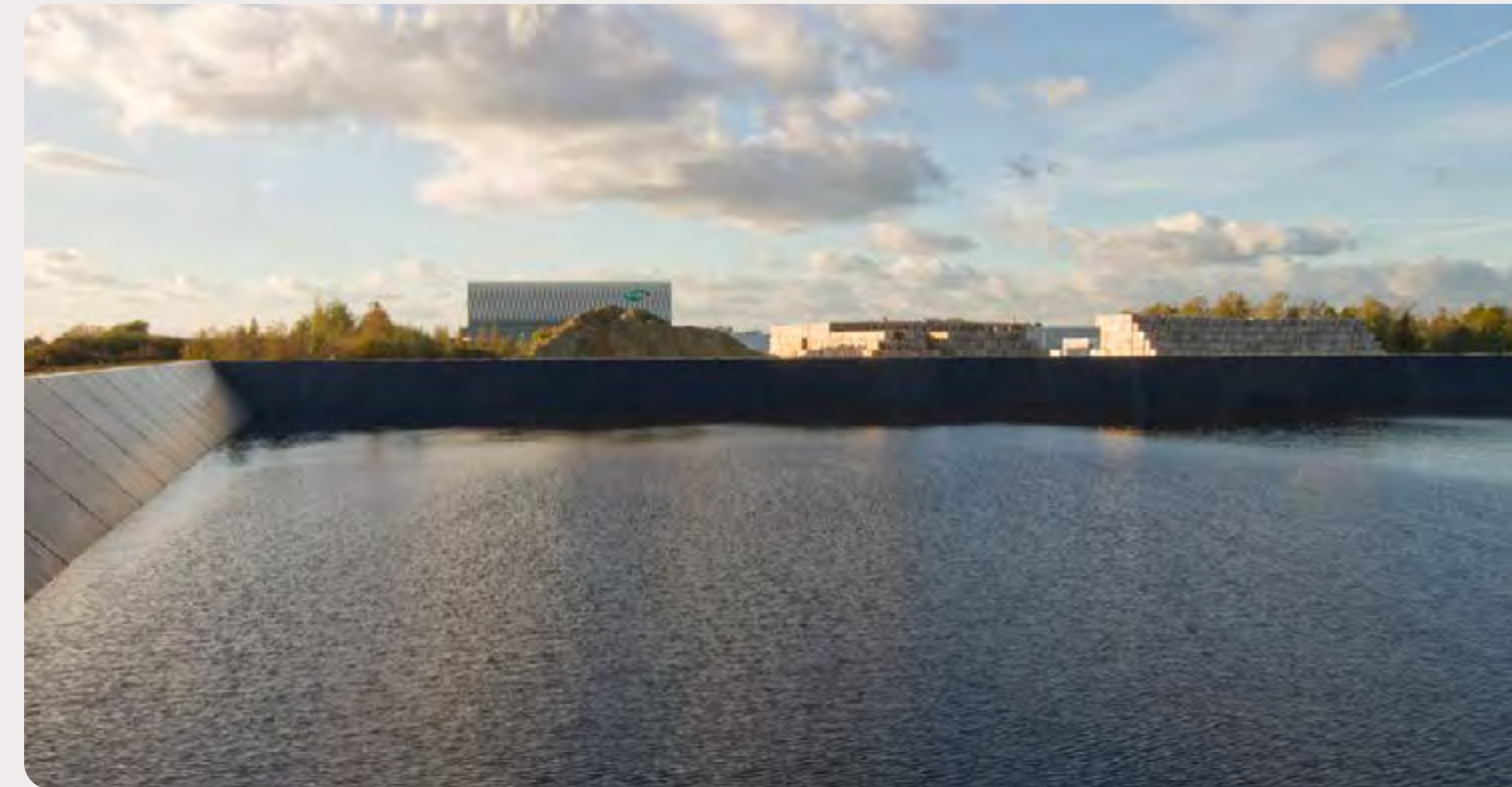
In Ardooie, the purified waste water from the Ardo site is pumped into a 150 million liter reservoir
